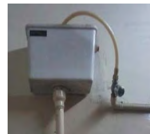
Fig. 3. Flush tank of conventional urinals
